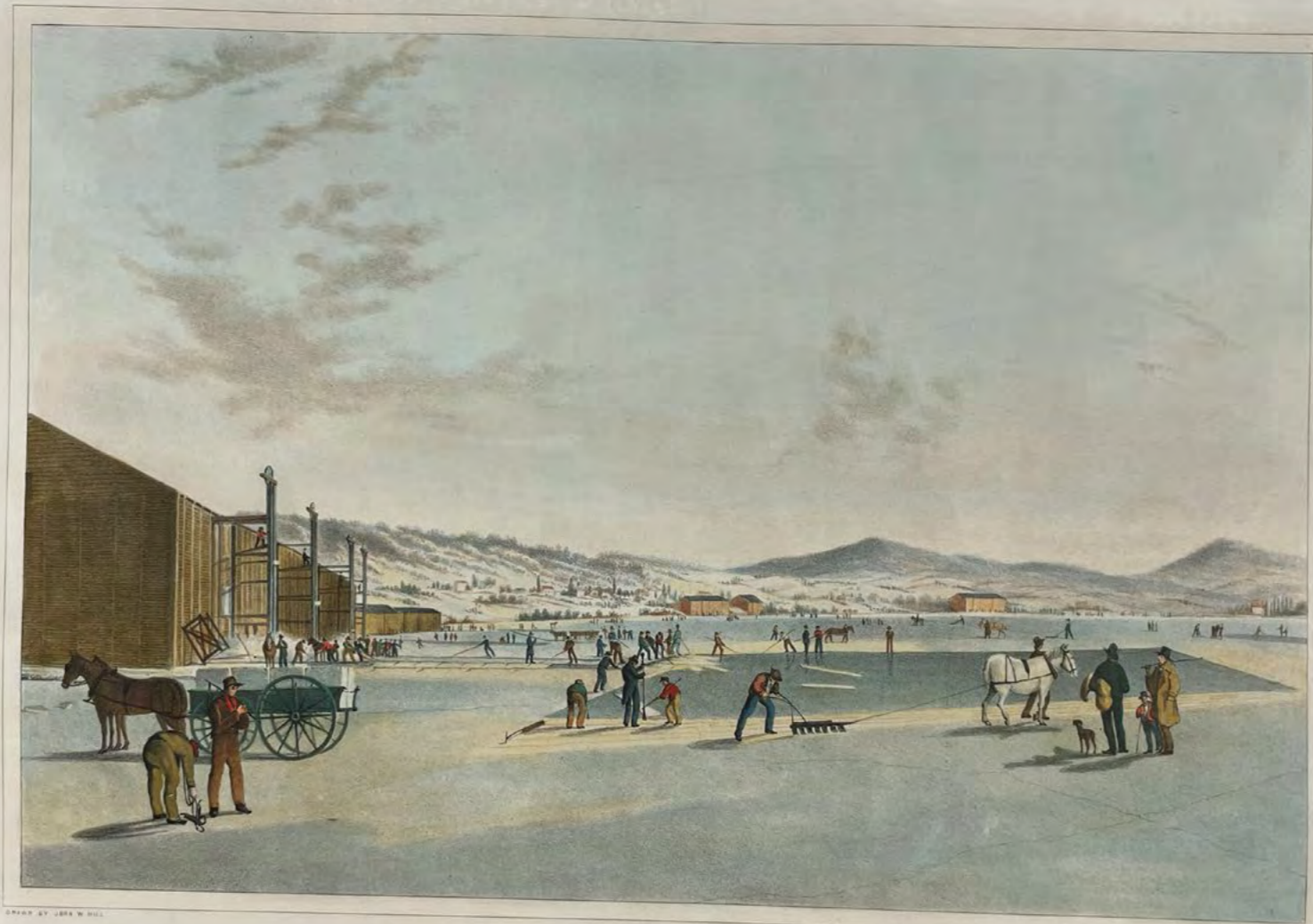
ROCKLAND LAKE - CUTTING ICE. VIEW FROM THE NORTH EAST.
